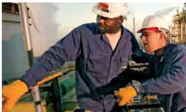
Sasol Infrachem employees working on a Sasolburg autothermal reformer.
