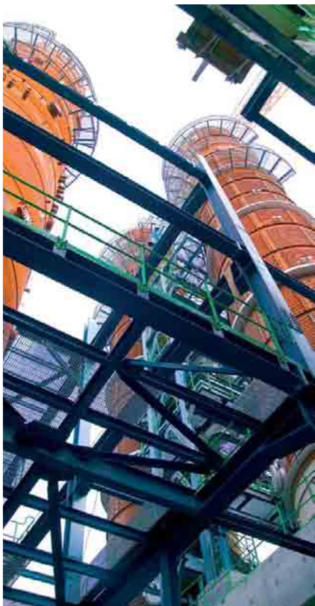
The Oryx GTL plant is one of the group's major new investments being executed with expert support from Sasol Financing.
