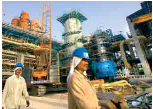
The Oryx GTL plant under construction at Ras Laffan, Qatar.
