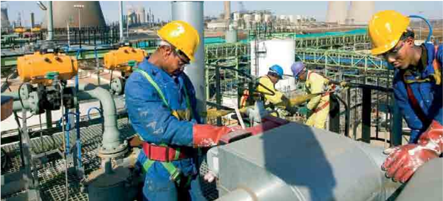
A new Sasol waste-recycling facility under development at Secunda in South Africa.
