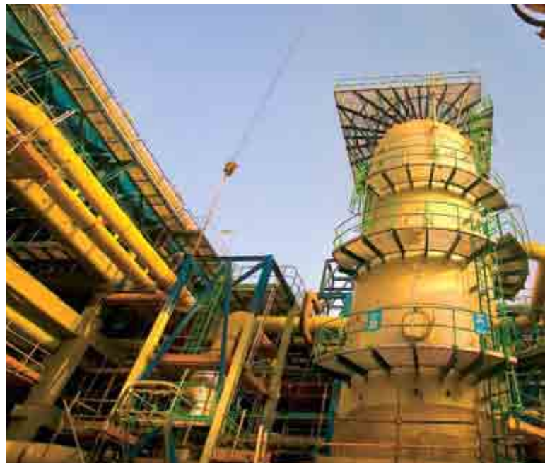
The Oryx GTL plant in Qatar will supply environmentally preferred synthetic diesel.
