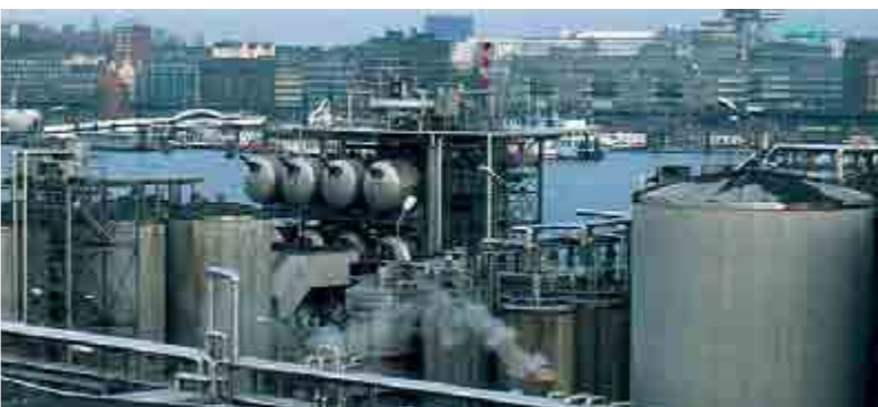
The Sasol Wax plant at Hamburg in northern Germany.
